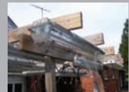
4. Place New LIRA Optically Clear Lens on fixture and latch closed.
