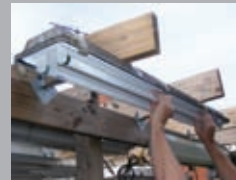
2. Attach a New Basic or Wide Reflector to the existing gear tray
